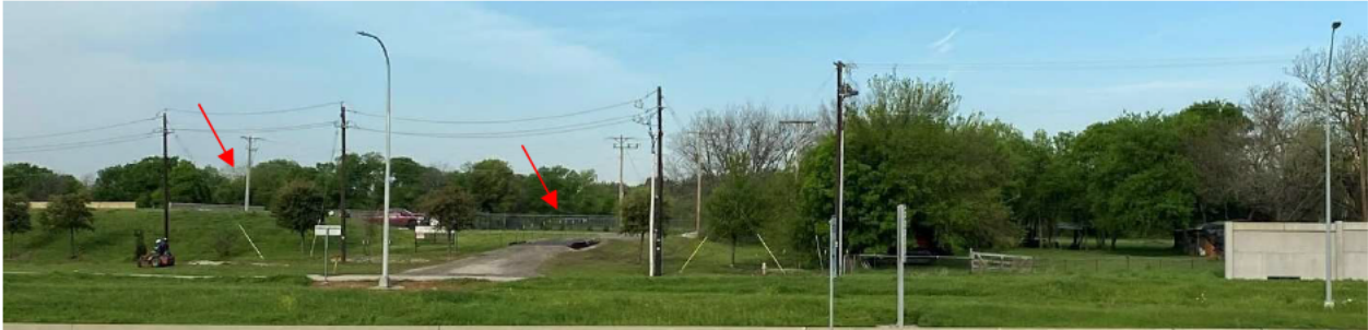
Fulson drill site and frac pond from South Watson Road.
