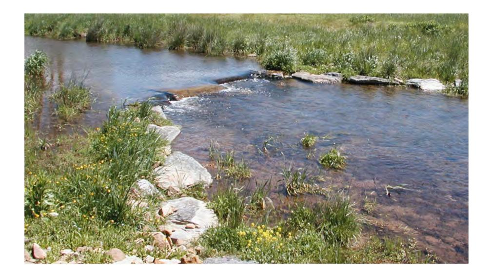
Figure 12. Example of a Constructed Rock Cross Vane
